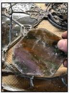
Once the glass restoration process was begun by Nathan from *Art Factory America*, the original stained glass was carefully removed from the deteriorated glass caming, with extreme care taken to retain as many pieces as possible for reuse. Any missing or broken pieces were replaced using close visual matches, sourced from multiple artglass vendors.
