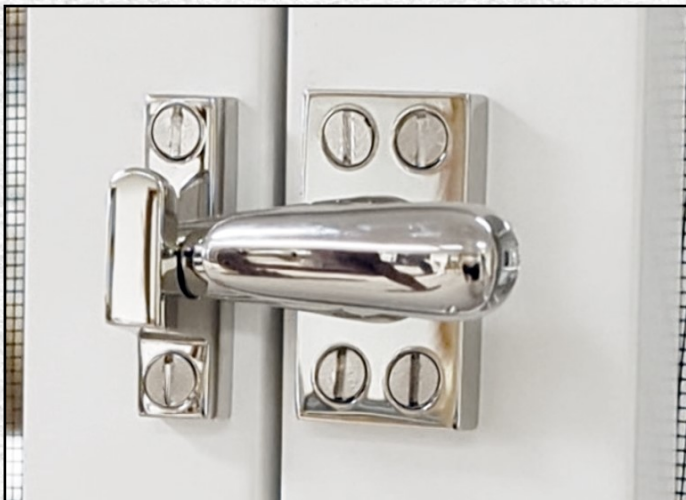
Detail of singlepoint locking screen latch (Polished Chrome Finish).
