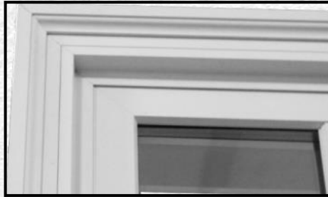
Closeup of Parrett applied aluminum brickmould casing.
