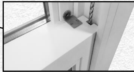
Detail of exposed sash chain and sash limit device.
