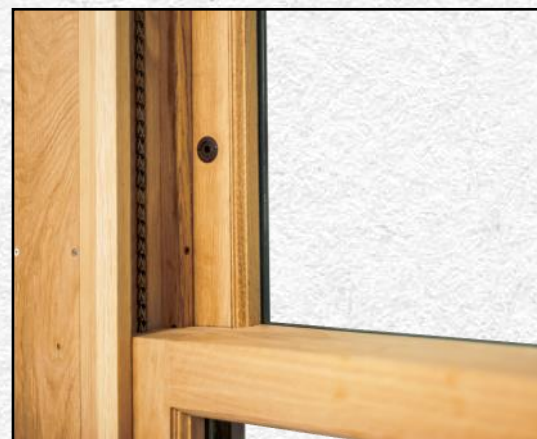
Sash chain and sash limit device are visible in this checkrail detail view.
