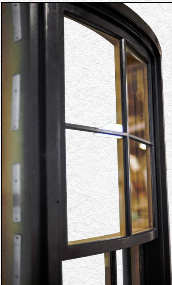
The contrast of the curved sash can be seen when compared to the angled TDL bars, and flat glass pieces as seen in the detail above and below.
